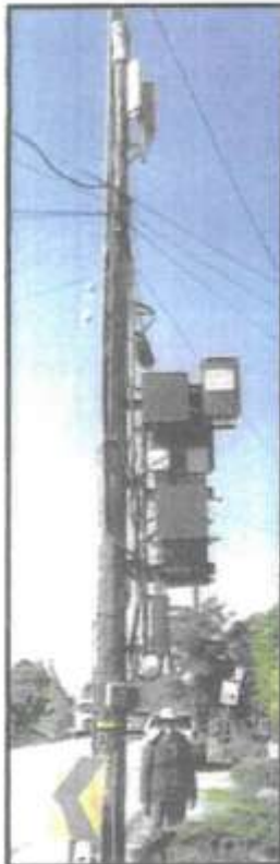
"An AT&T Mobility Small Cell on an existing utility pole in Oakland."
